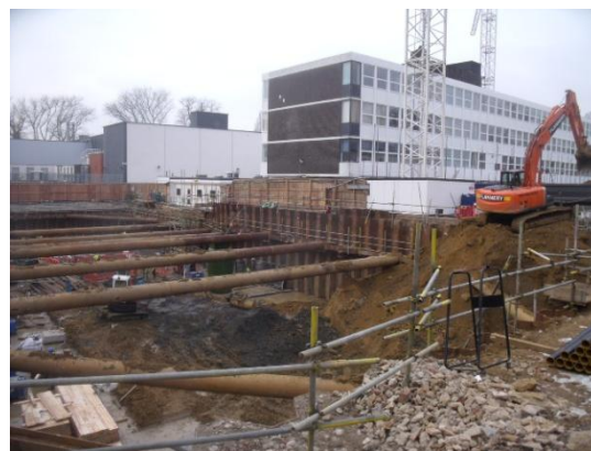
Foundation pit for new Kennedy Institute
